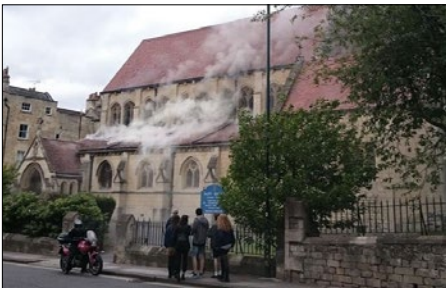
A remarkable shot of the fire at St Mary's. Photo: Sam Cox, www.nowbath.co.uk
