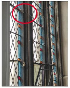
The western-most window in the south gallery needed urgent stonework repairs where one of the mullions (circled) had cracked right through — a common problem in older buildings, we're told, caused by the rusting and expansion of the metal horizontal members holding the glass in place. You can see an area of "blown" stone lower down on the same mullion caused by the same thing.
