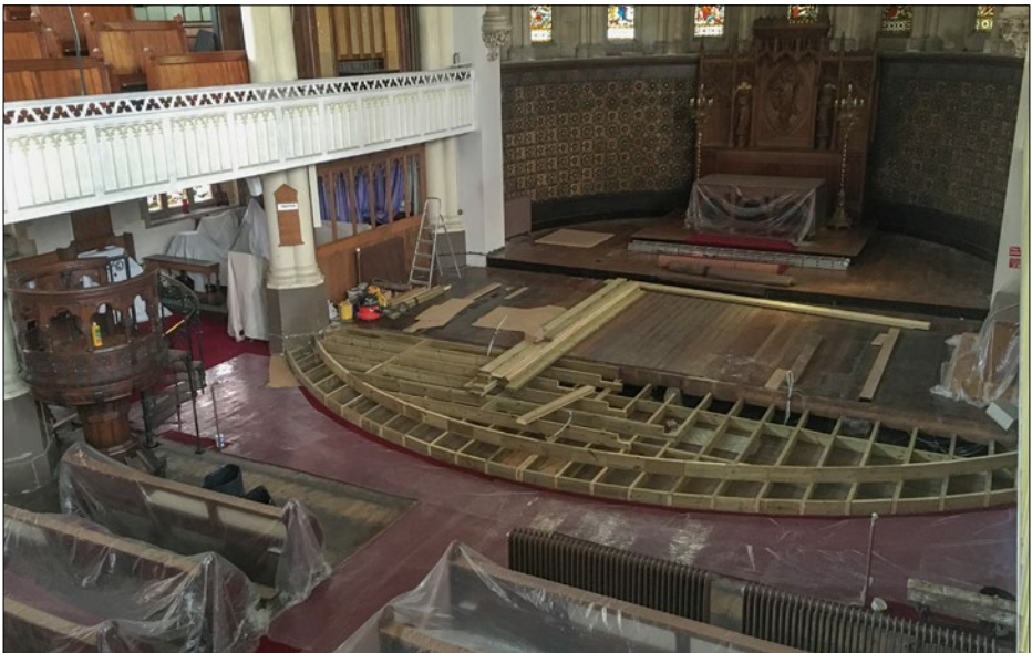
The new curved chancel extension is taking shape.
